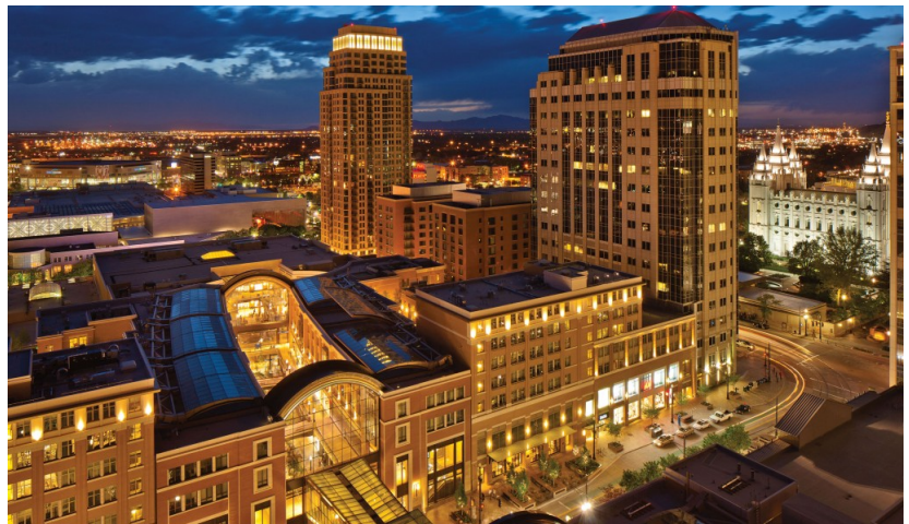
City Creek Center has a retractable glass roof to accommodate Salt Lake City winters. The lighted Mormon Tabernacle can be seen at the far right. (William Tatham, SWA Group)
